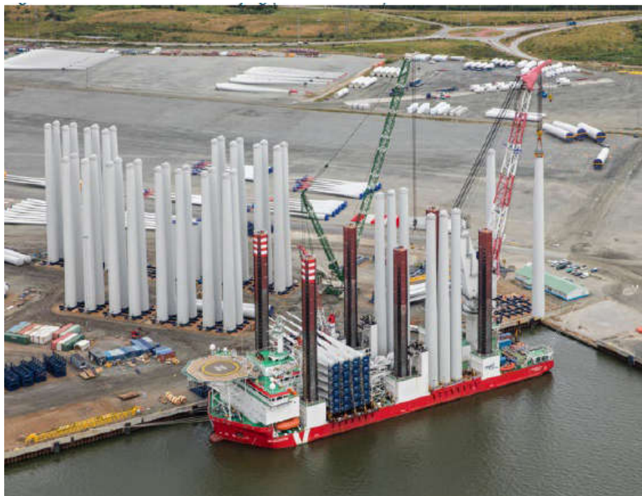
Figure 2: Wind turbine components loading activities to WTIV
